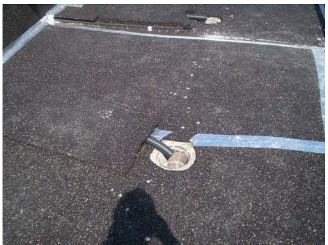
Fig. 6: Fleece as protective layer
