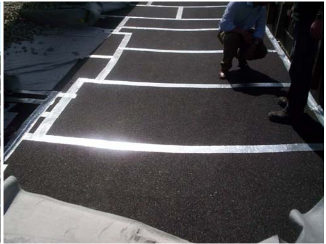
Fig. 4: Gluing the joints with special adhesive tape
