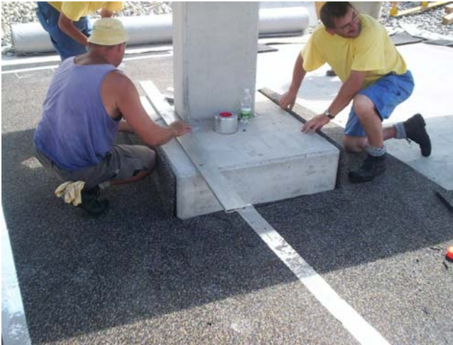
Fig. 9: Cutting out around pillars
