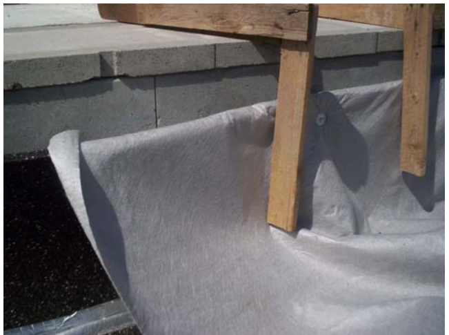
Fig. 6: Fleece as protective layer
