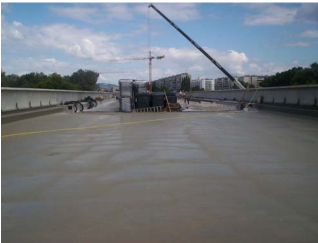
Abb. 1: Sealed concrete surface
