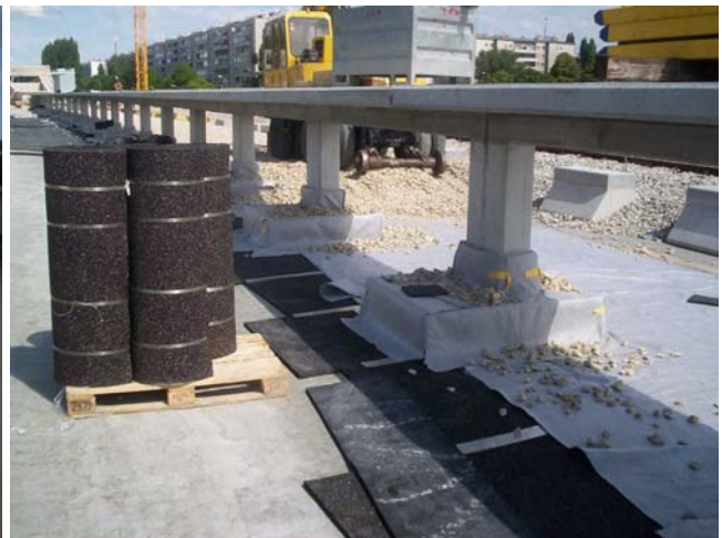
Abb. 2: Delivery of product rolls DAMTEC ® KRAIBURG USM Sub Ballast Mat on a pallet
