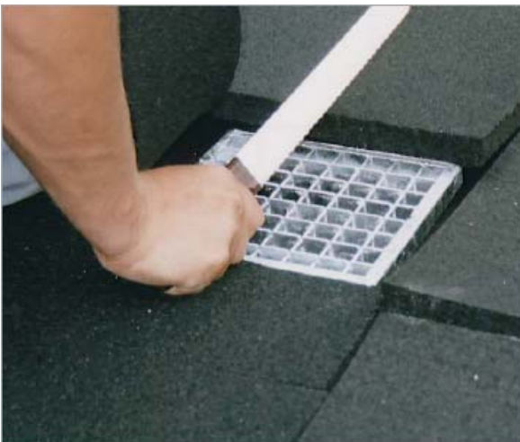
Fig. 10: Cutting out the Sub Ballast Mat for drainage areas
