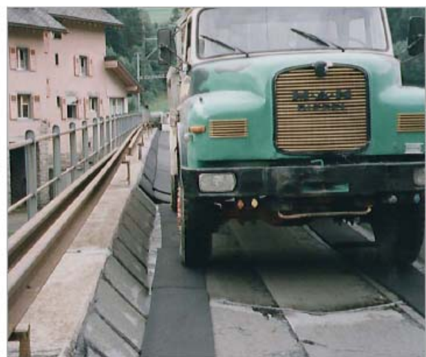
Fig. 7: Transporting the Sub Ballast Mat to the installation point
