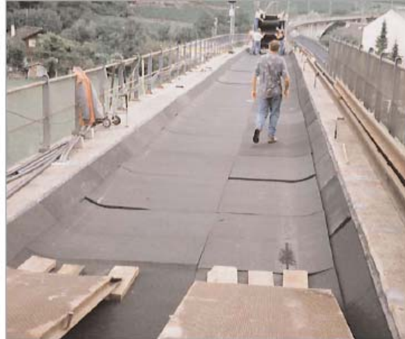
Fig. 9: Laying the Sub Ballast Mat
