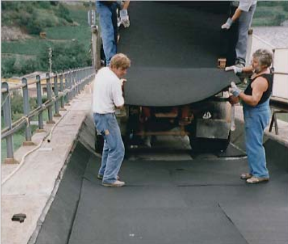
Fig. 8: Laying the Sub Ballast Mat
