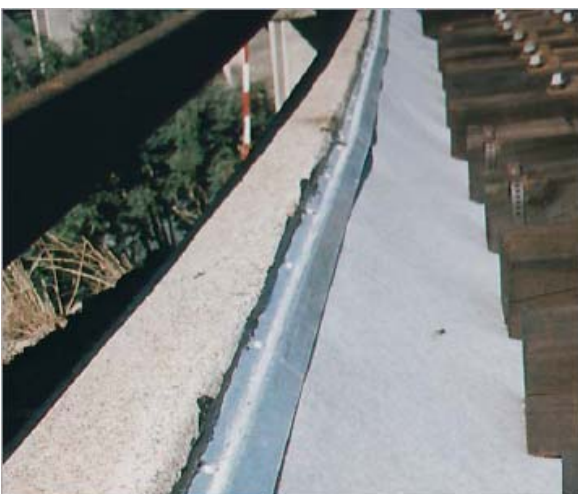
Fig. 12: Fleece and cover sections as protection against dirt and gravel abrasion
