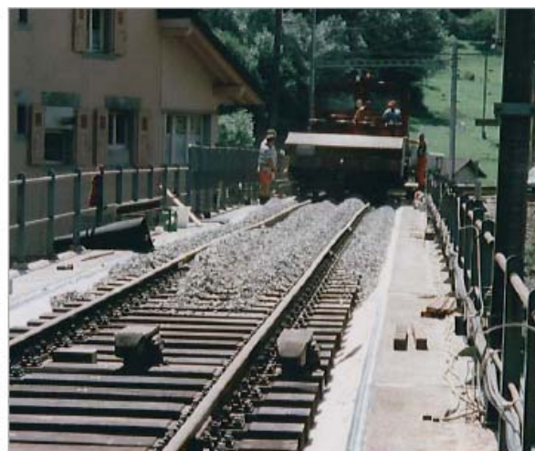
Fig. 13: Laying the Sub Ballast Mat
