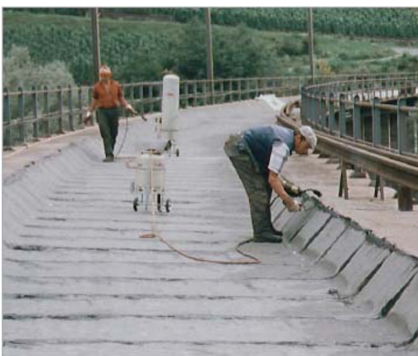
Fig. 6: Welding the watertight covering layer
